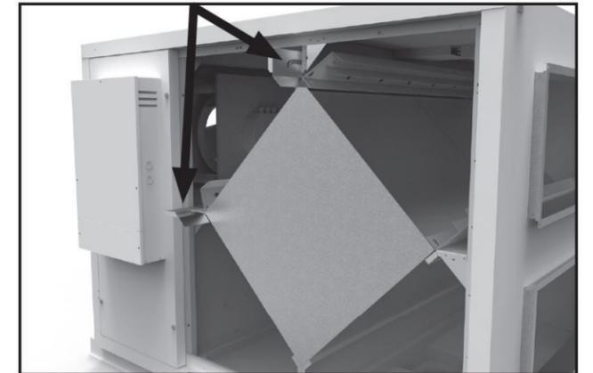
**To install the clean Core and Filters.**
